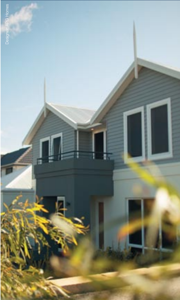
Western Australia builder APG has pioneered lightweight construction in upper storeys.
