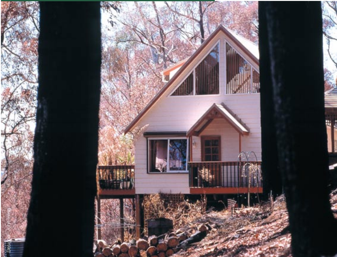
In Victoria, charred vegetation surrounds this home, which survived a bushfire intact. It was clad in HardiPlank® from James Hardie.
