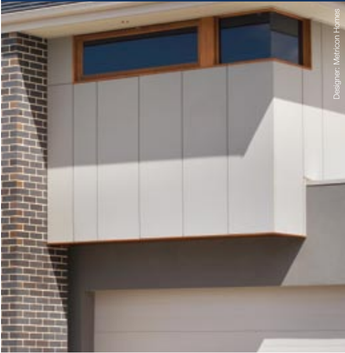
Scyon™ Matrix™ cladding butts up to brickwork in Metricon's new display home.
