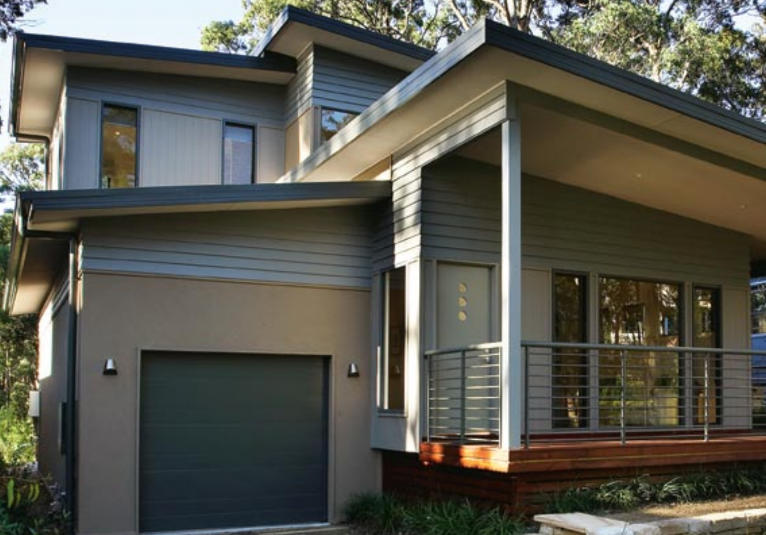
This home at Murrays Beach in New South Wales uses Linea weatherboard, Axon cladding and HardiFlex® eaves lining.
