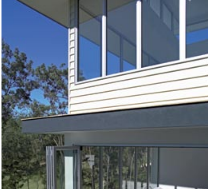
This home at Brookwater golfing estate features Scyon™ Linea™ weatherboard, HardiPanel® compressed sheets and HardiTEx® system.
