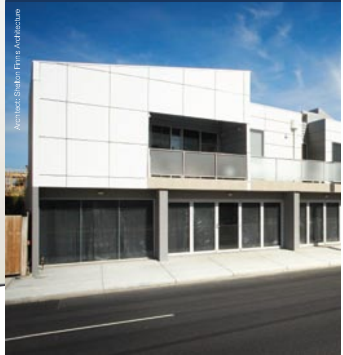
Scyon™ Axent trim, Matrix™ and Axon™ cladding, and Linea™ weatherboard feature in this development in Melbourne.
